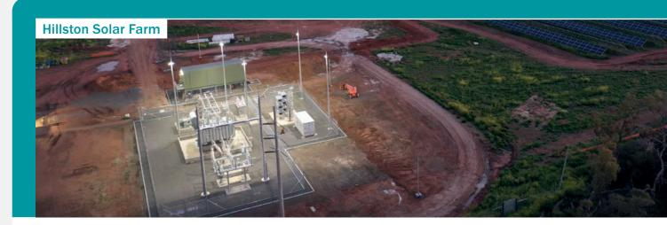
The Hillston 85 MW Solar Farm, located near Hillston in central NSW, was connected to the Essential Energy network and fully commissioned in March 2022, via the 132/33kV Hillston zone substation. It can power up 48,000 homes, generate 23,500 MWh of clean energy annually, and reduce 160,000 tonnes of CO2 emissions per year.
