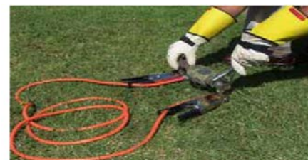
Bridging out of water meter
