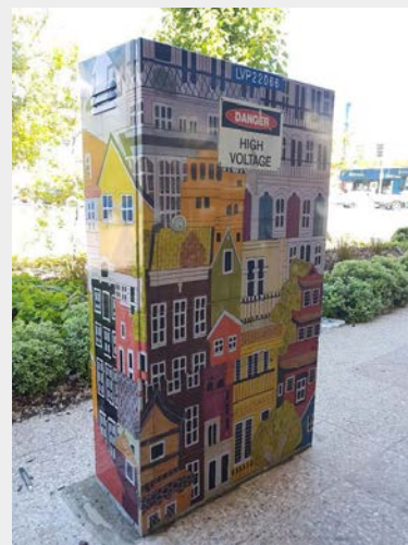
A community partnership in Goulburn aims to inspire local artists and reduce graffiti on Essential Energy assets.
