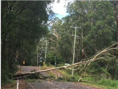
Network damage was sustained following storms in Coffs Harbour on Christmas Day.
