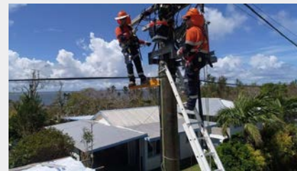
Essential Energy field employees working to restore power in Tonga.
