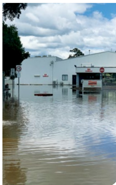
Inundation of our Cowra depot during the November 2022 flood.
