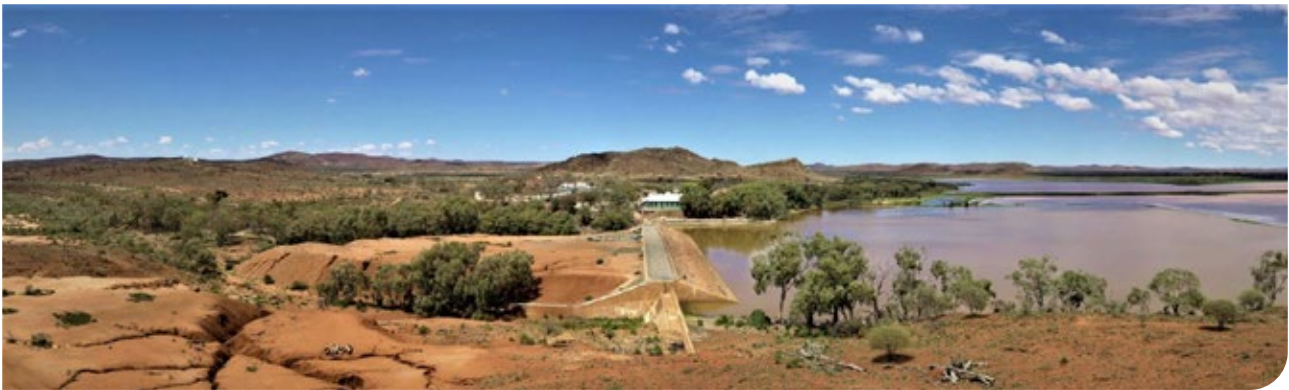
Stephens Creek Reservoir – part of Essential Water’s network of dams, reservoirs, pumping stations, treatment plants and pipelines.
