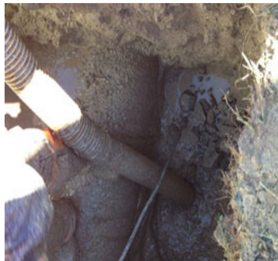
Hydro excavation in progress
