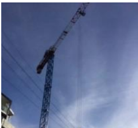
Figure 16: Overhead powerline clearances must be adhered to when operating any mobile plant or equipment, including cranes.
